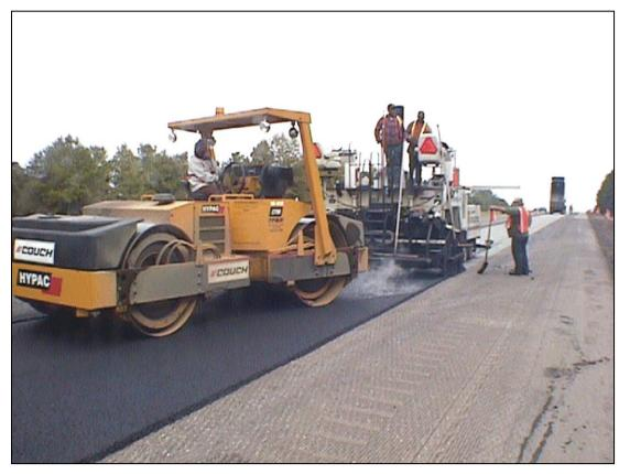
Good compaction limits entry of air and slows oxidation
